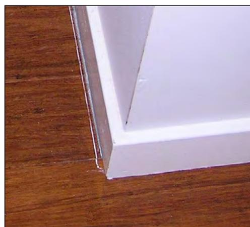
Also with floating floors the first of these two photos shows unevenness in the floor surface of this floated floor due to insufficient expansion allowance. This introduces excessive vertical movement when walking on the floor and can often introduce squeaking. The second photo indicates where length expansion in this bamboo floor has begun dislodging the moulding around the door frame.
