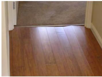
*Floating floor uneven due to insufficient expansion allowance*
