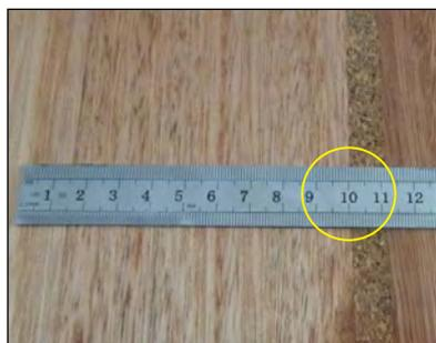
*Cork expansion joint in solid timber floor*
